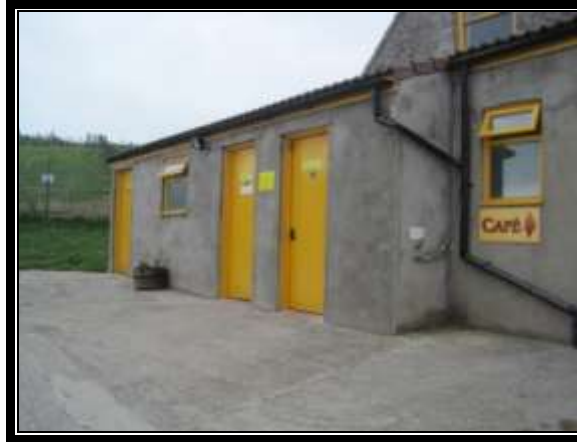
Disabled toilet cubicle (far left)
